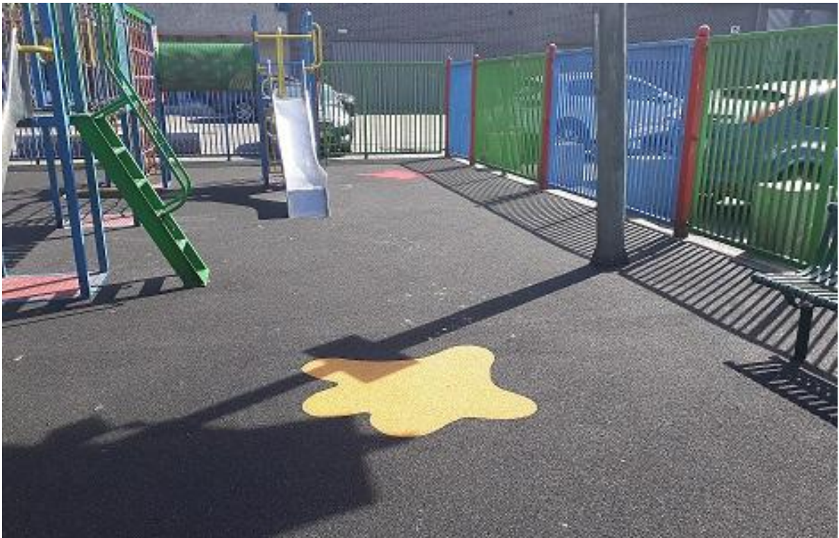
Upgrade works to playground at Liberty House now complete.
